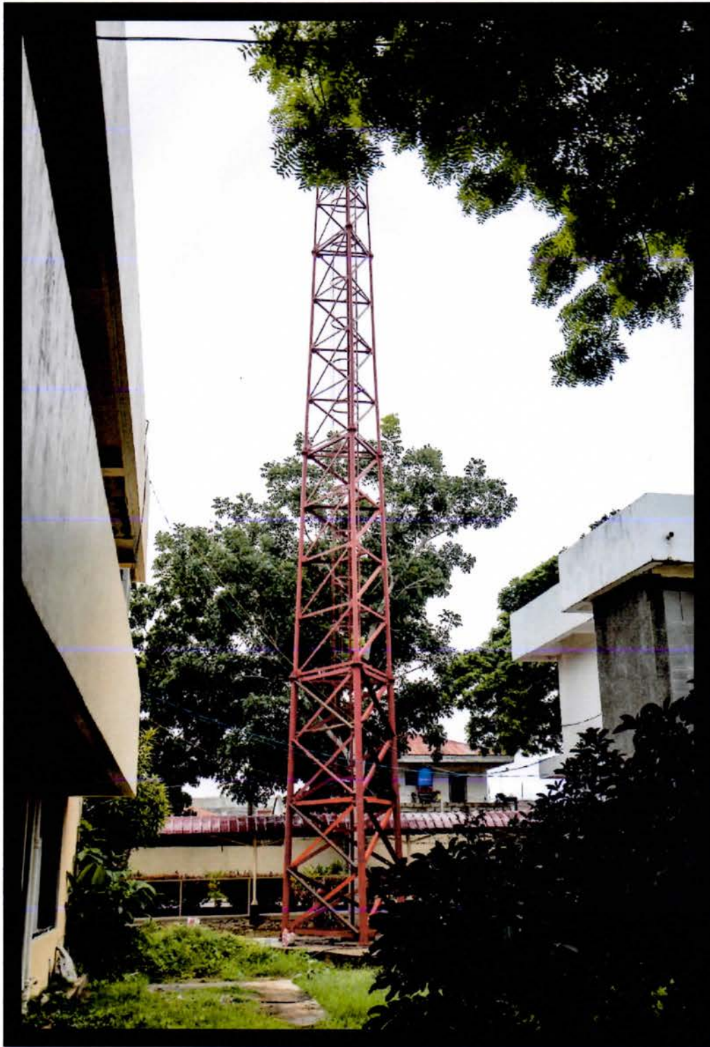
Construction of Galvanized 3-legged 80-foot Ground Based Tower
